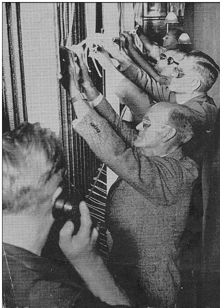
J.W. Vines and T.H. Harvey prepare to pull the heat coils to start the new service.
